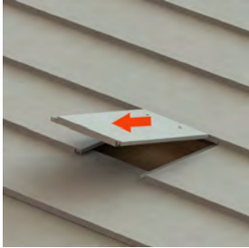
1. Remove the tile and locate the rafter.
