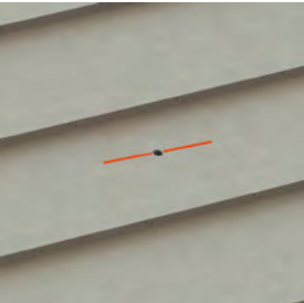
6. Carefully drill a hole through the tile using 1/2" drill bit.
