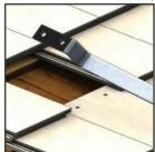
2. Insert the two (3/16" or 5/16") bolts through EPDM washers and the flat tile hook and apply fresh compatible sealant to the base.
